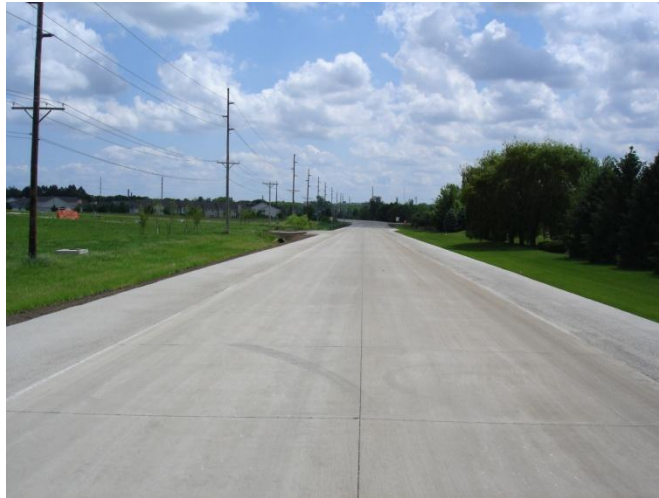
FIGURE F-6 Closed-course looking south from z-configured road tubes
