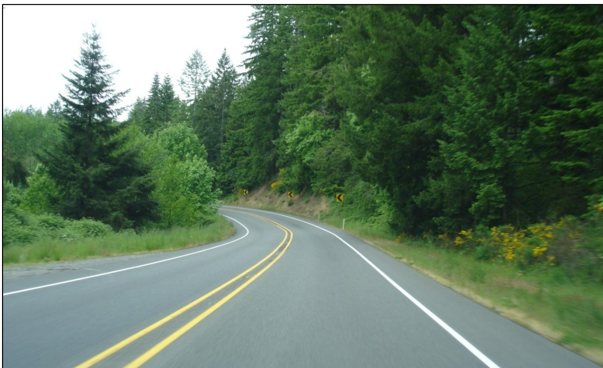
FIGURE 1-1 Rural horizontal curve on State Highway 510 in Washington outside of the Nisqually Indian Community with paved shoulders and chevron alignment signs
