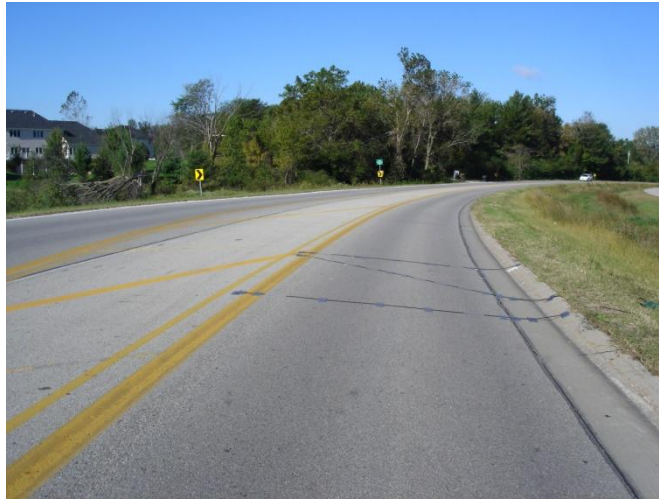
FIGURE G-11: Sta. A at point of curvature
